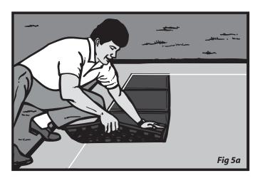
As the tiles are being installed each tile will need to be fitted as tightly as possible to the adjacent tile. This is normally done by using a rubber mallet or the heel of your foot to "kick" the tiles tight or snug.
