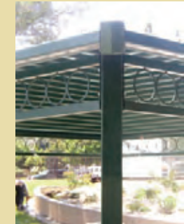
Close-up view circle pattern lattice and the pergola's steel slats
