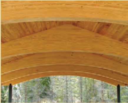
Laminated Curved Beam ceiling with 2"X6" Southern Yellow Pine Tongue & Groove roof decking
