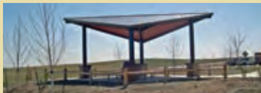
Model 8124SM Custom 24' Steel Beam Peaked Square shelter with 8" square columns and standing seam metal roof. Masonry by others.
