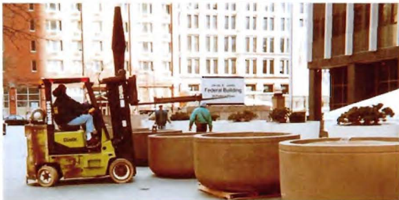
Installation of RP-Planters by Petersen Mfg.
