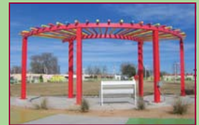
Rear view of Santa Fe Pergola.
